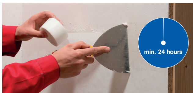
Figure No. 6: Reinforcement tape - technological break at least for 24 hours follows.
