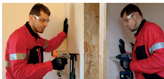
Figure No. 4: Mounting of the boards with clamps or screws.
