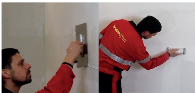
Figure No. 7: Top sealing; Firestop finish sealant polishing (if necessary).
