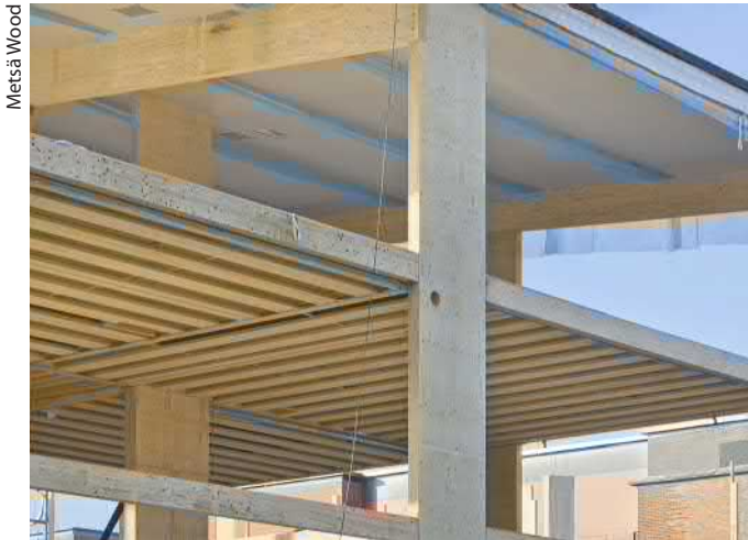
Figure 2.20. LVL open box slabs of intermediate floor constructions in multi-storey buildings.
