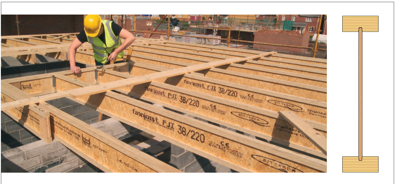
Figure 2.94. Wooden I-joist with LVL flanges.
