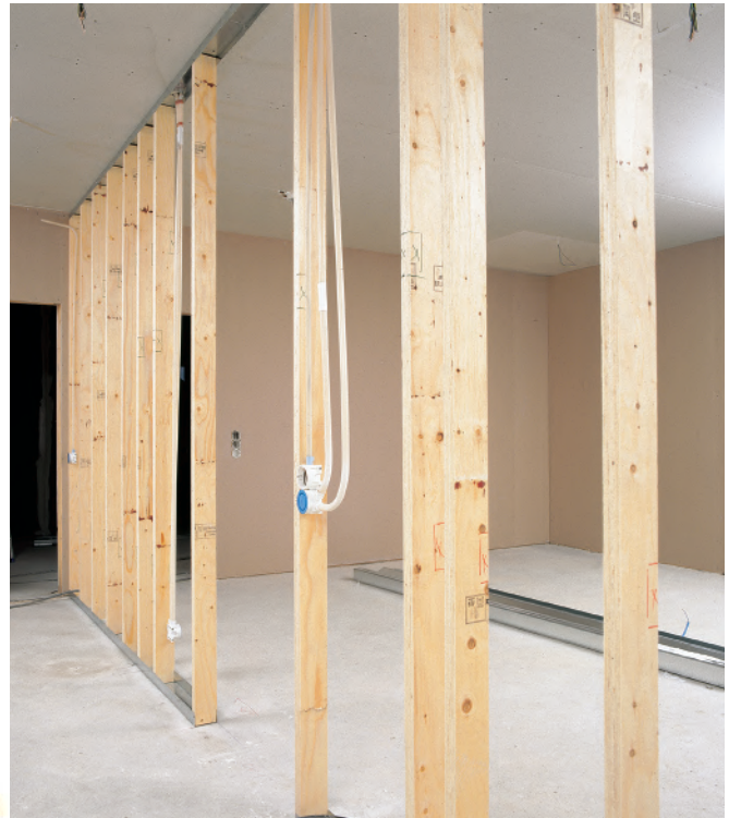
Figure 1.59 LVL-P wall studs.
