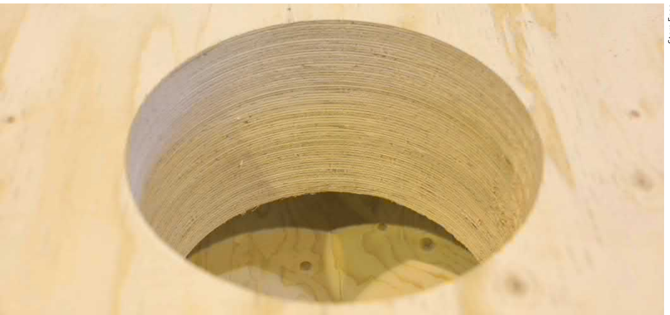
Figure 1.50. Hole in an LVL beam.
