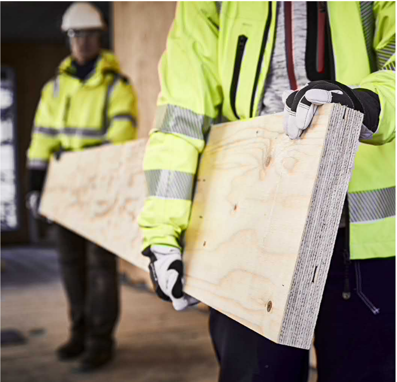
Figure 3.1. Handling of LVL beams
