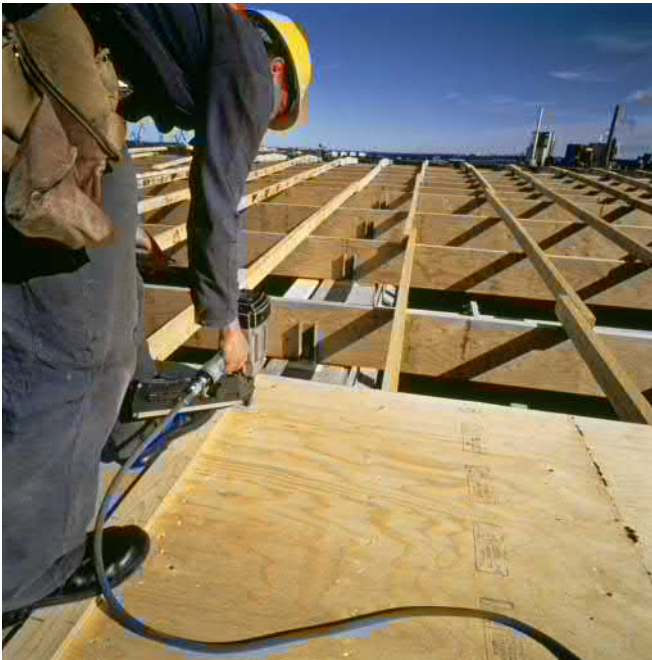
Figure 2.45. Installation of LVL-C roof panels.
