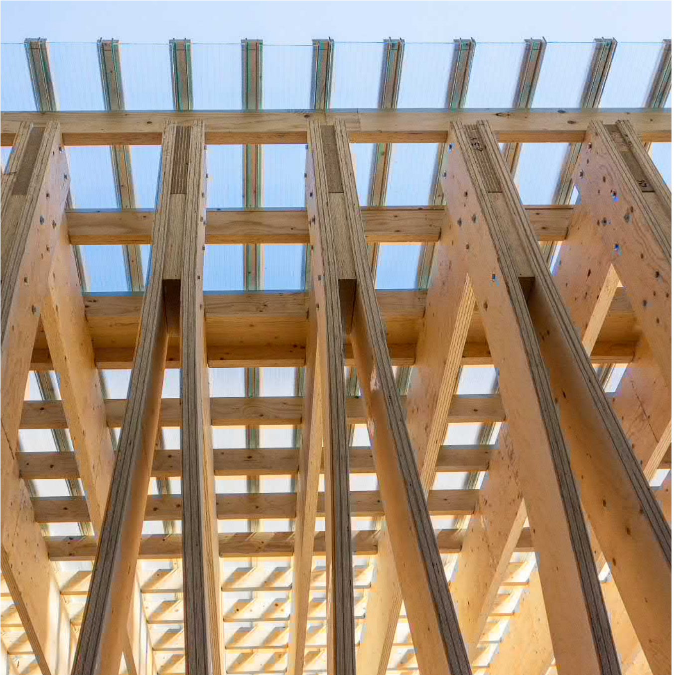
Figure 5.1. LVL connections.
