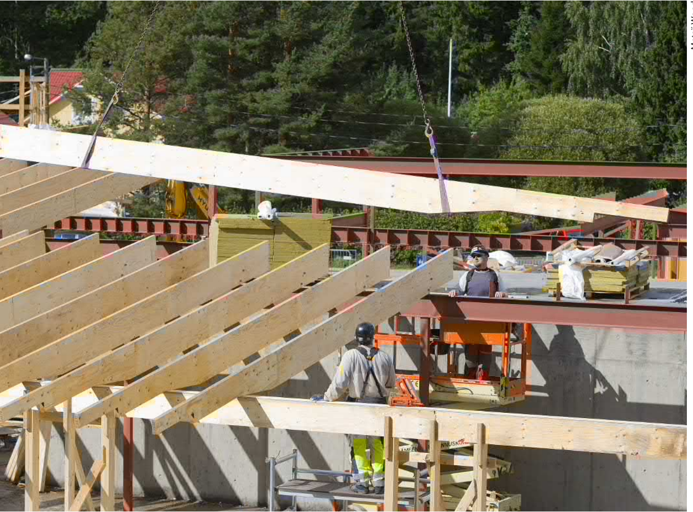
Figure 1.49. LVL-P roof beam cut to special shape.
