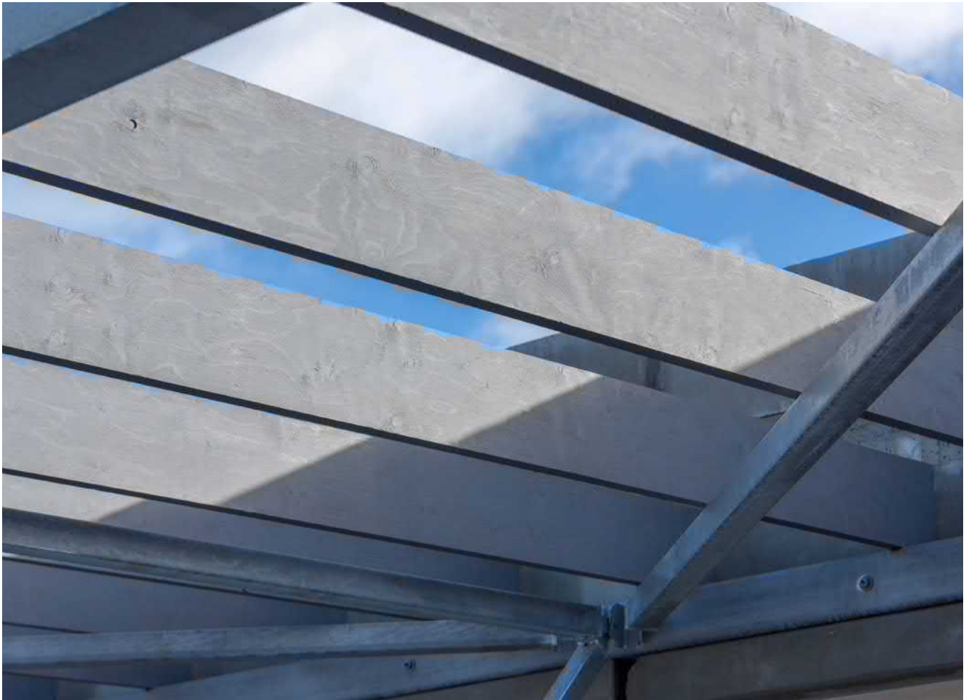
Figure 1.66. Coated surfaces of LVL beams.
