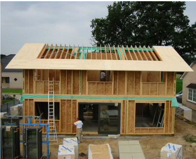
Figure 2.47. Eaves and roof overhangs from LVL-C panels.
