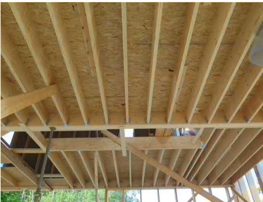
Figure 2.2. LVL-P joist floor structures.
