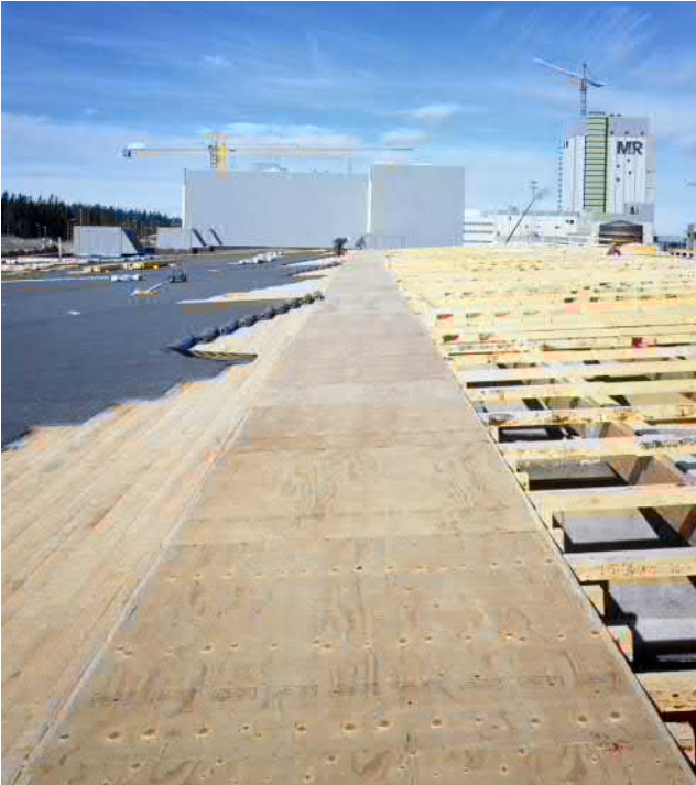
Figure 1.4 LVL-C roof panels.
